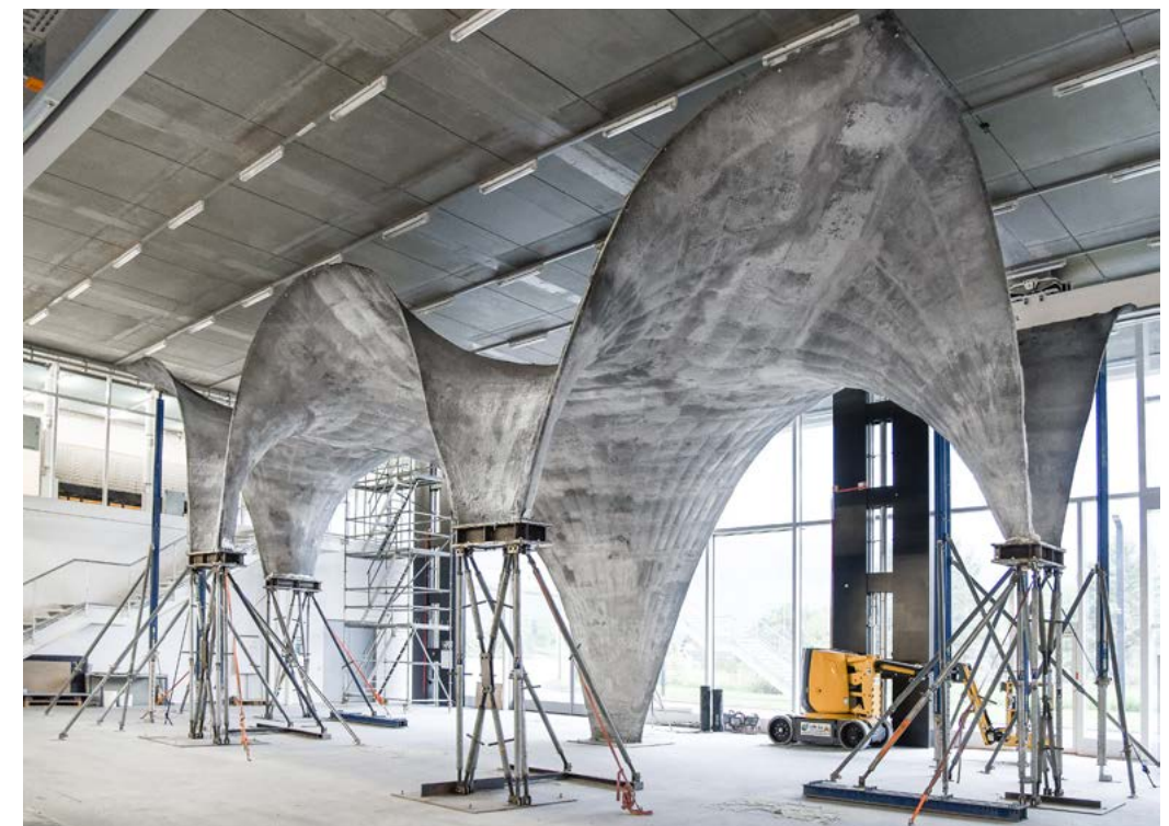
Fig 5, Construction prototype for ultra-thin concrete roof Zürich, 2017 Photo: Block Research Group / ETH Zürich
