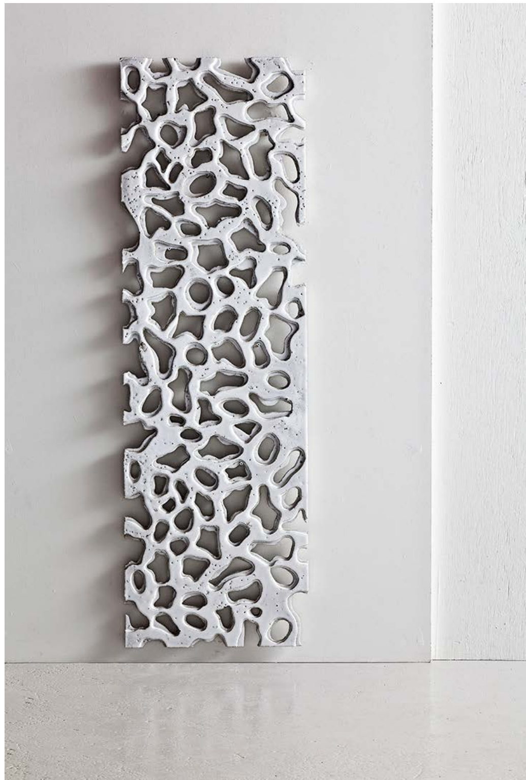
Fig 10, A façade panel for a mounted façade solution in specific ceramic glazed concrete by Anja Margrethe Bache. Copenhagen, DK 2013 Photo: Ole Akhøj
